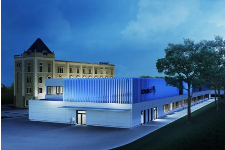
New Premises Novaled, south view technical center and mill from Königsbrücker Straße
