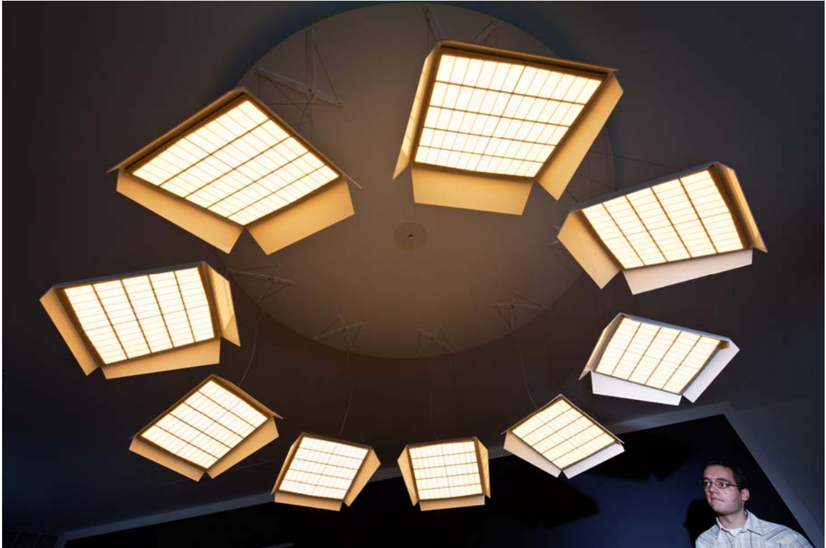
Abb2: The OLED-tiles and their arrangement are optimized for a homogenous illumination of exhibits on display.
